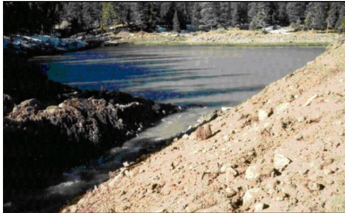
Initialization of the breach in the embankment dam 8
